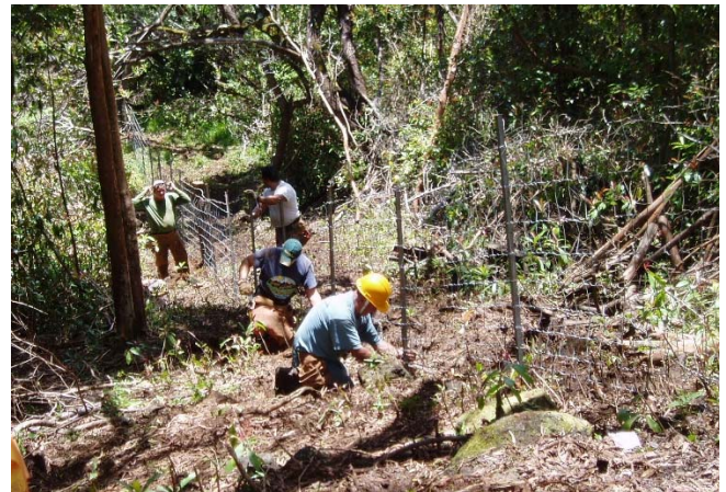
Ungulate fencing installation
